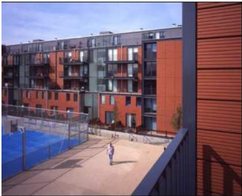
Figure 19 Mixed modular and panel building using light steel framing at Lillie Road, Fulham Courtesy, Feilden Clegg Bradley
