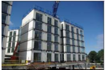
Figure 22 Modular units supported by a podium Courtesy, Fusion Building Systems Ltd.
