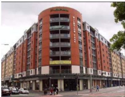
Figure 20 Typical podium structure in which seven storeys of residential units are supported on a composite frame below
