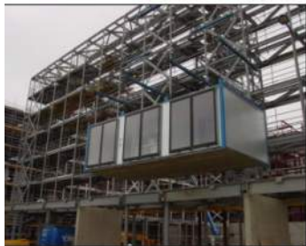
Figure 21 Installation of modules behind external steel framework at MoHo, Manchester Courtesy, Yorkon and Joule Consulting Engineers
