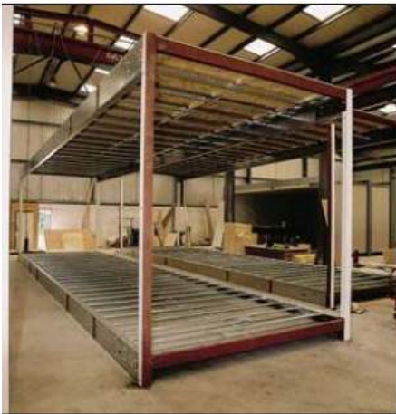
Figure 11 Primary steel frame used in an open-sided module Courtesy, Kingspan Off-Site and Modular UK
