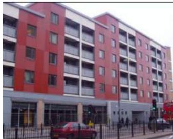
Figure 23 Mixed use of stabilising frame and modules in a residential project in Shadwell, East London Courtesy, Rollalong
