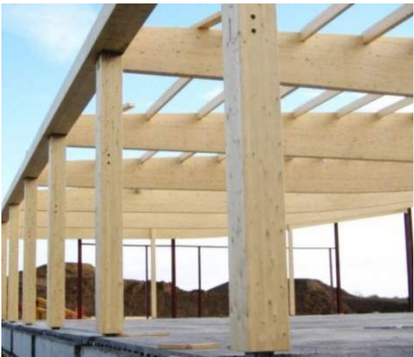
Post & Beam Construction (Glulam)
